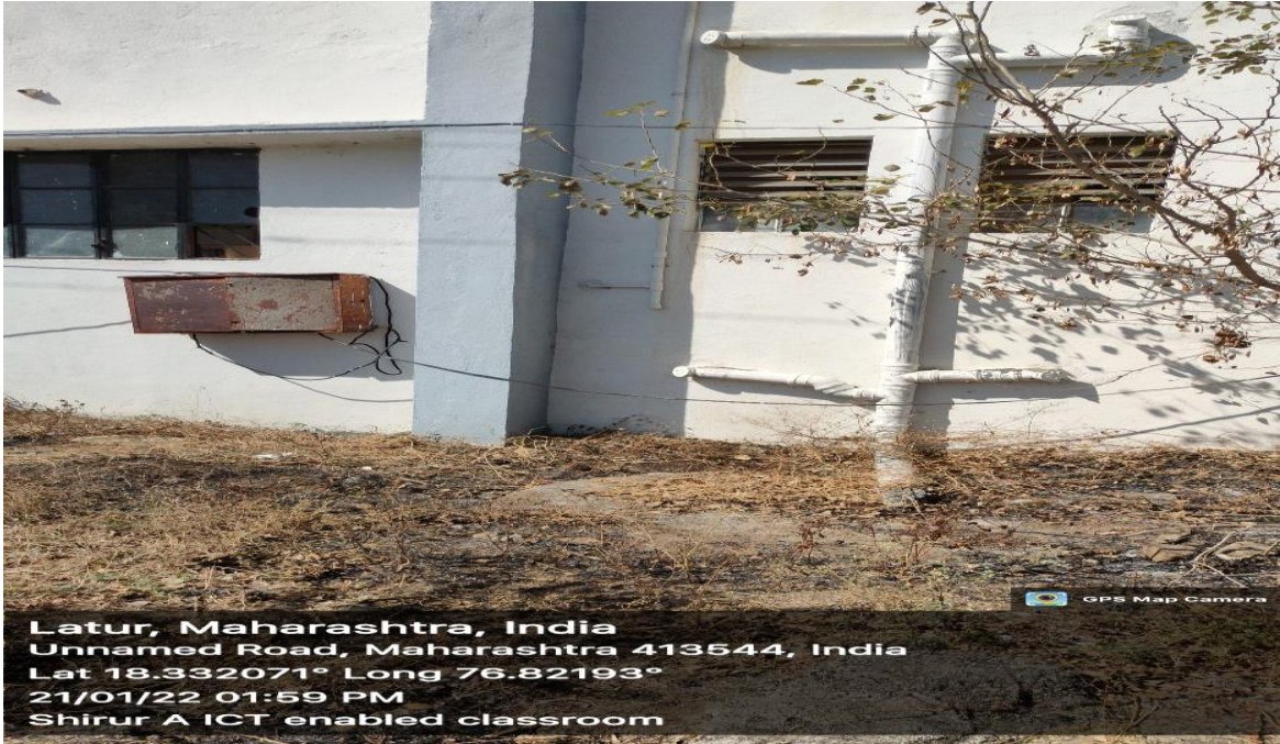
Bore Well facility
