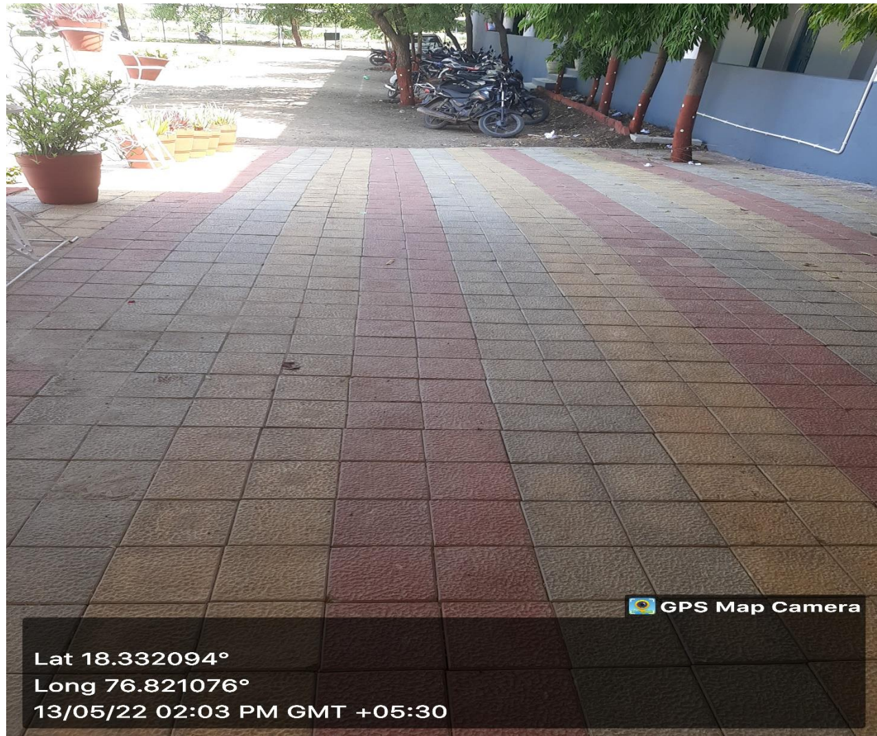
Ramp for differently Abled Person
