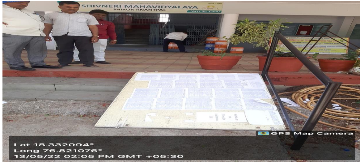
Ramp For Differently Abled Person
