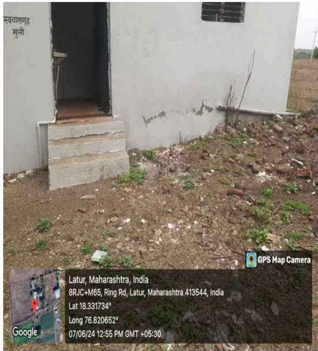
Washroom facility for Girls Students
