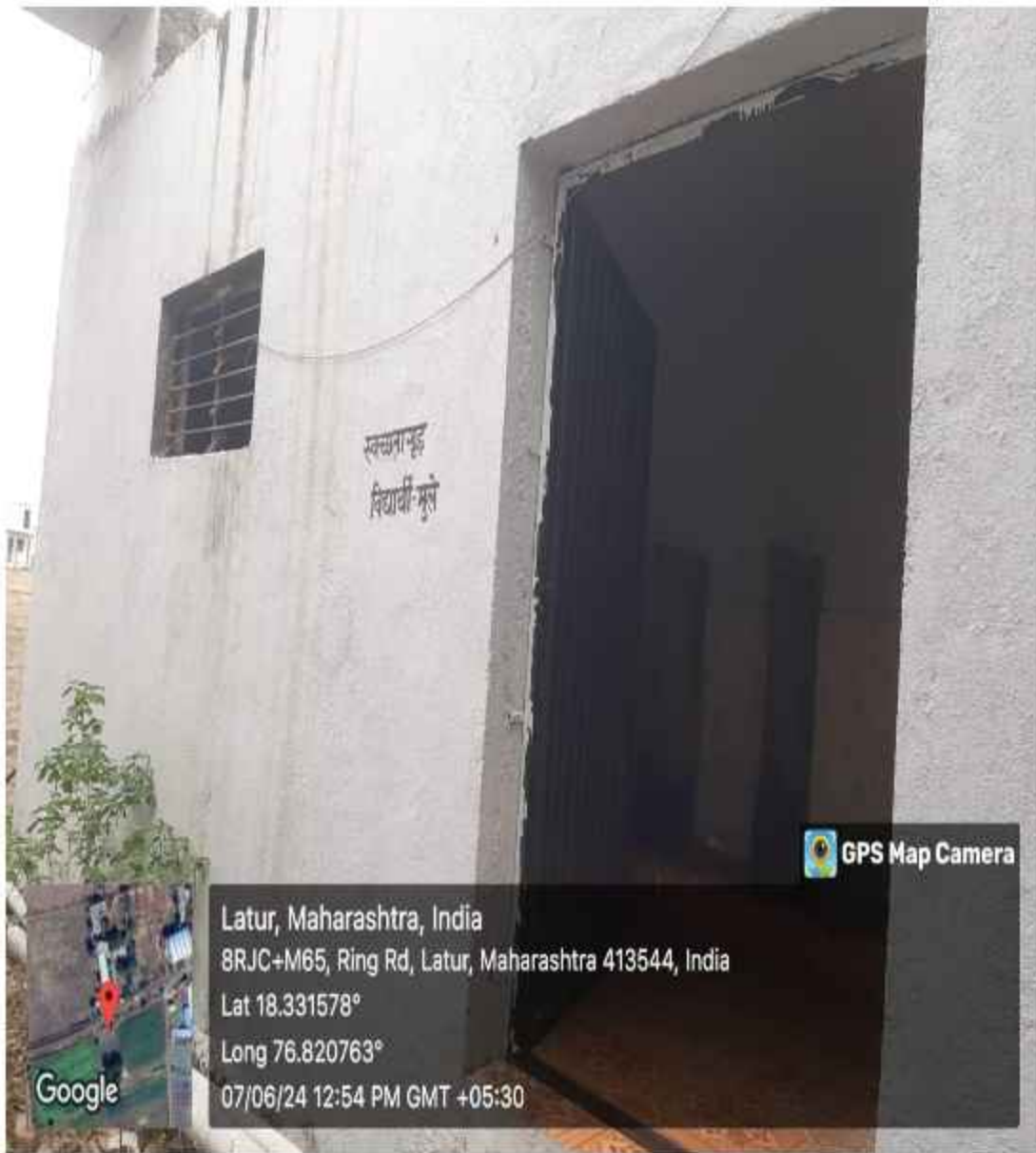
Washroom Facility For Boys
